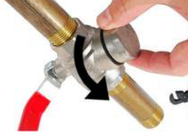
Fig. 7 - taking out the strainer
